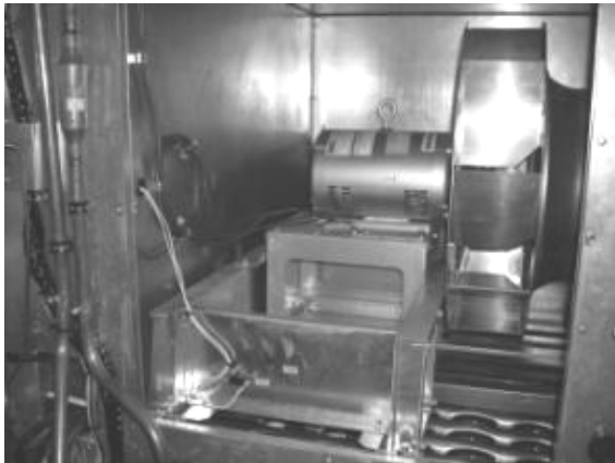
Figure 37 - 6-25 and 30 ton Supply Fan
