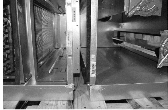
Figure 11 - Connect Sections
