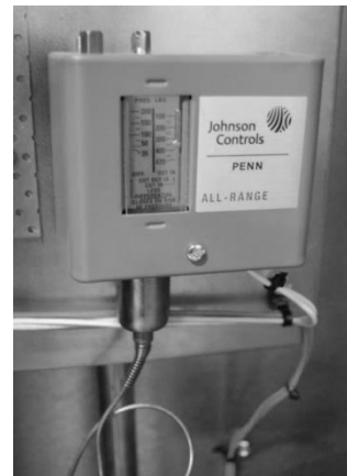
Figure 7 - Adjustable Fan Cycling Switch
