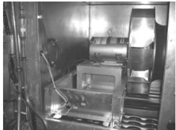
Figure 39 - 11-25 and 30 ton Supply Fan
