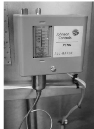
Figure 7 - Adjustable Fan Cycling Switch
