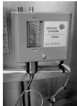
Figure 7 - Adjustable Fan Cycling Switch
