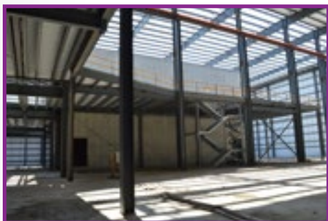
Open Testing Area Under Construction
