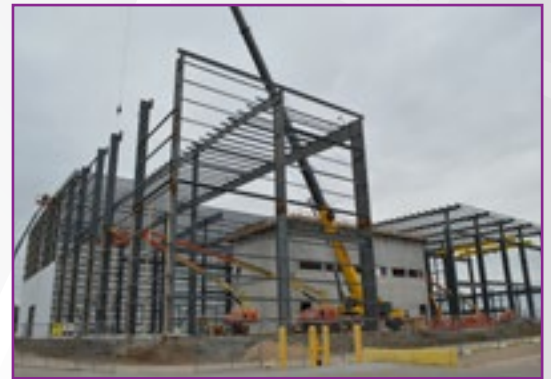
Structural Steel Work
