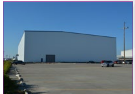
Exterior Wall and Roof Completed
