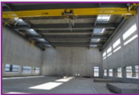
Test Chamber Interior Under Construction
