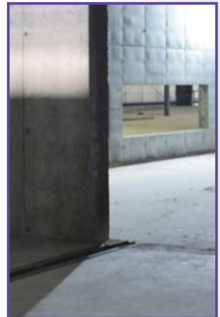
Sound Chamber Walls are 12 Inches Thick Concrete
