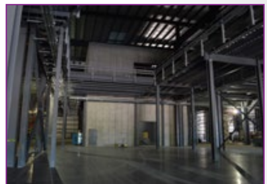
Interior Construction Underway
