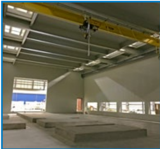
540 ton Test Chamber Interior
