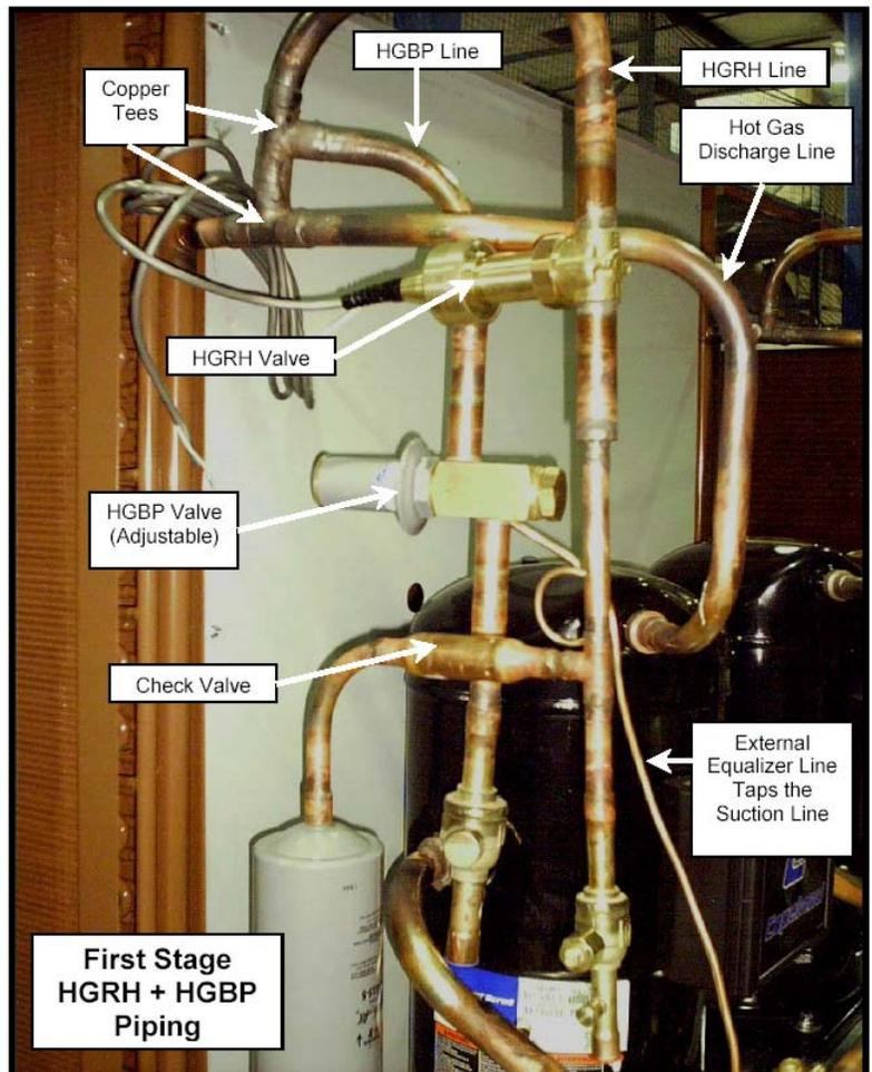
Figure 10.2, HGRH with External HGBP Piping
