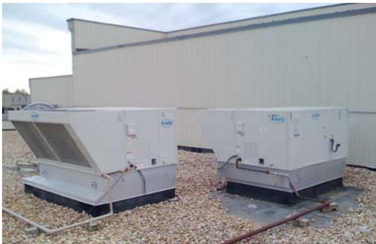
Equipment with variable capacity scroll compressors can control supply air temperature and space temperature more accurately than equipment with standard compressors because the compressors can modulate their capacity almost instantaneously to match the load. This is because the pulse control signal has only a short duration.
