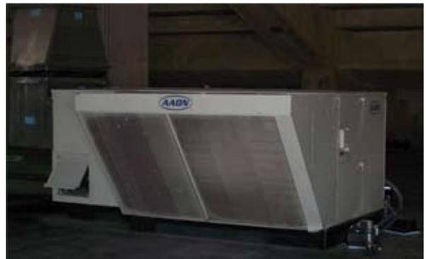
*"The units on the locker rooms had to function in two separate modes. This separate mode function was made very easy" explains Ed Adams, of Chet Adams Company, "with the controls and AAON having a feature to turn off the energy recovery wheel and exhaust fan as well as closing the outside damper."*
