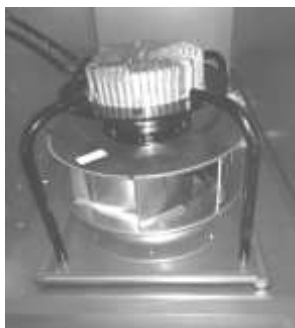
Figure 21 - SB Series Supply Fan
