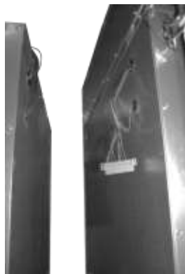
Figure 10 - Low Voltage Quick Connect
