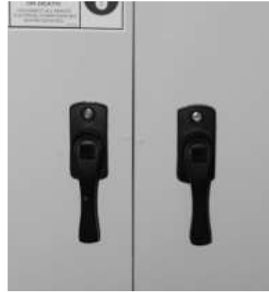
Figure 1 - Lockable Handle
